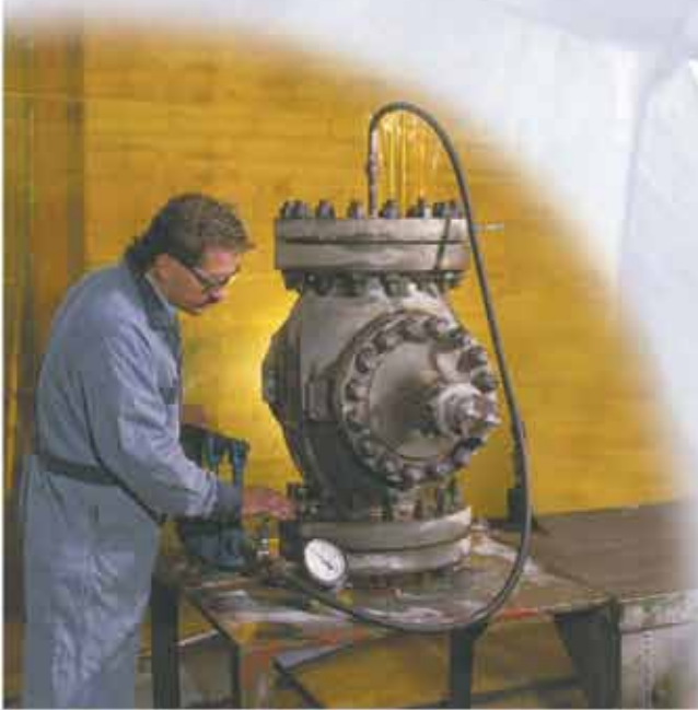
◀ Valve Inspection, Rebuilding & Testing
